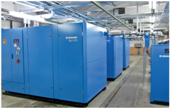
All from a single source: planning, installation, pipework and cabling.
